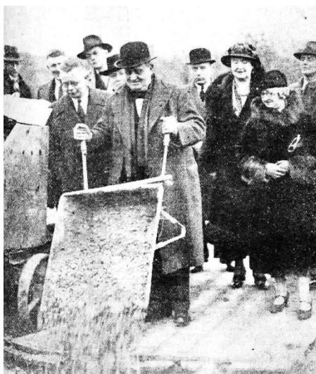
Mr Wise laying the first concrete and steel foundations for the new picture house at Keynsham.
