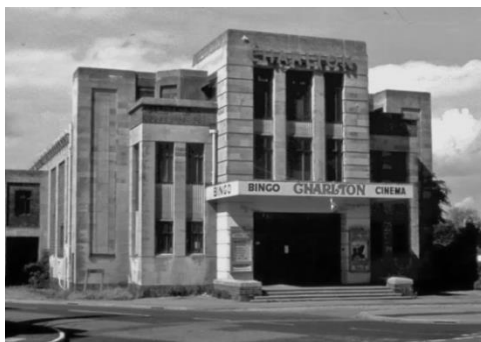
No longer a cinema, the Charlton Bingo Hall on 24 July 1997 prior to demolition.
