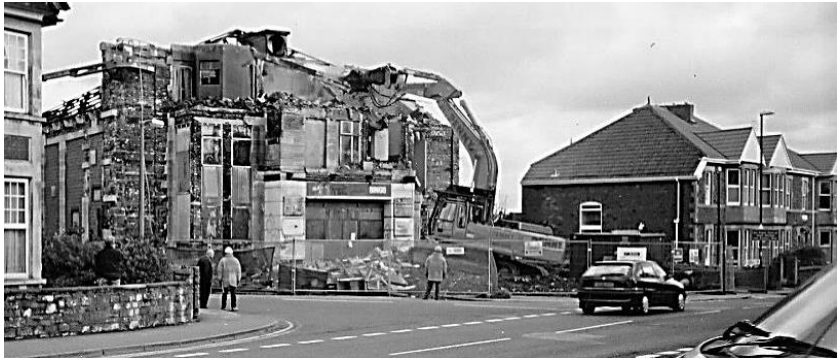
The end of the Charlton on 13 April 2005 and below right, the flats which have replaced it.
